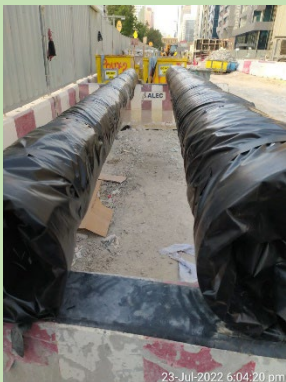
DI Pipe Rapping and Sleeve Installation
