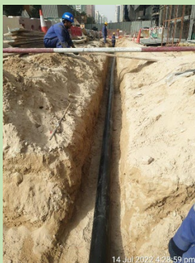
HDPE Pipe Laying and dressing
