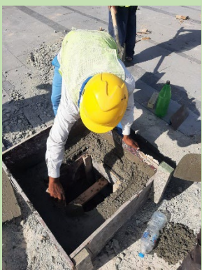
Finishing work for Pull Box
