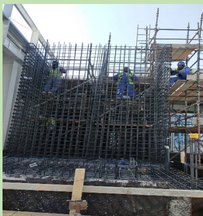
Wall Cage preparation work at ICAD
