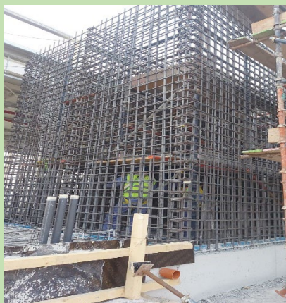
Raft Foundation, Steel Cage for wall
