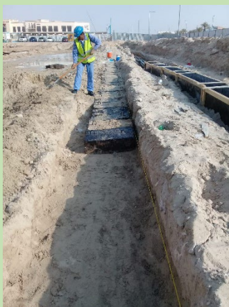
Precast Protection Slab Casting work for services
