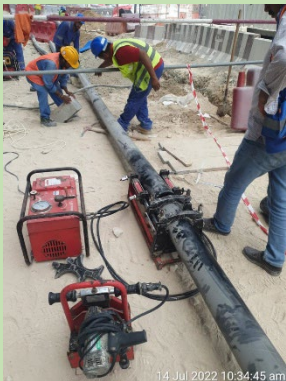
HDPE Pipe Welding
