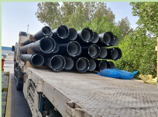
DI Pipe 300mm pipeline work for Potable Water Works
