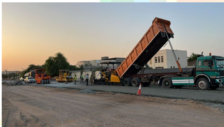
Asphalt Laying and Compaction
