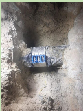
DI 300 Potable water Emergency Work
