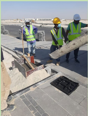
Pull Box concreting
