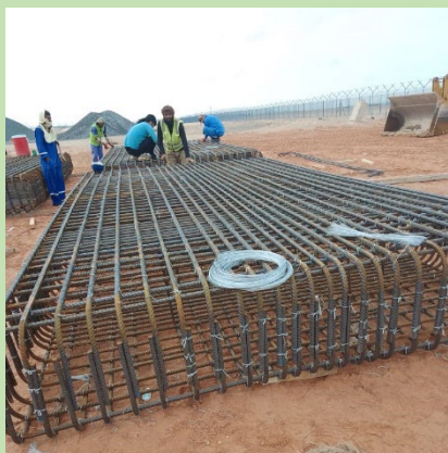
Foundation Cage Preparation at Borouge-4 Project
