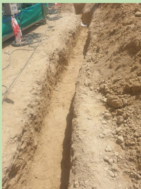
HDPE Pipe 160mm pipeline trench for laying pipeline
