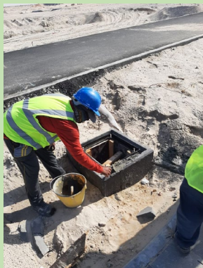
Pull Box Finishing work
