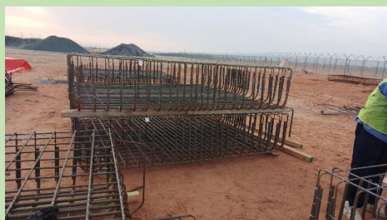
Foundation Cage Preparation at Borouge-4 Project
