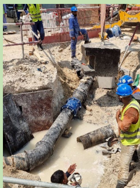
DI 300 Potable water Connection & Tie-in
