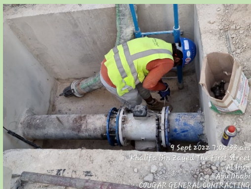
Flow Control Valve Assembly
