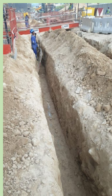
DI Pipe 300mm pipeline trench for laying pipeline
