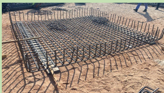
Foundation Cage Preparation at Borouge-4 Project
