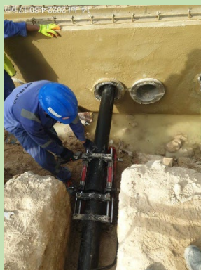
HDPE Pipe Welding inside the trench (Narrow space)
