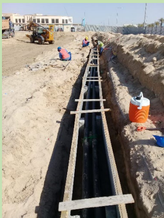
Etisalat Duct 2W, 4W, 6W and 8W Duct Construction
