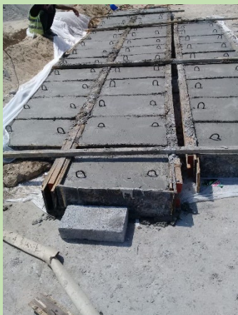
Precast Protection Slab Casting work for services
