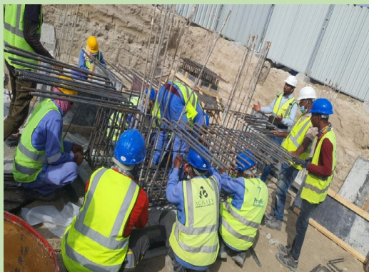
Pile Cap Construction
