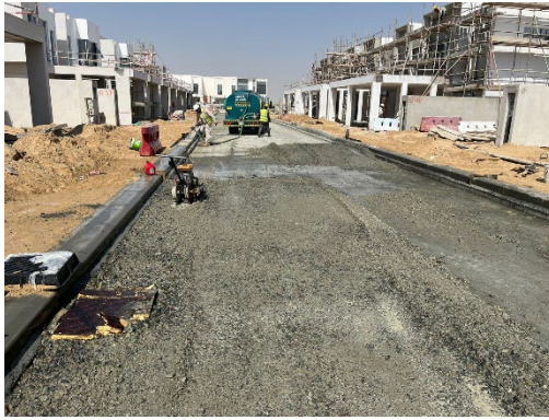
Road Base compaction
