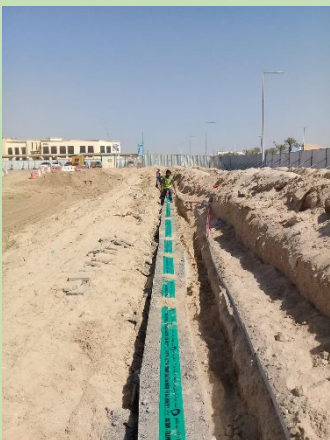
Electrical Service Protection work
