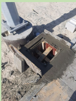
Pull Box Finishing work
