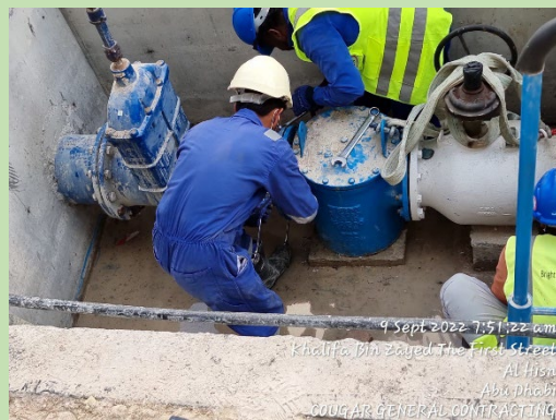
Gate Valve Chamber Assembly
