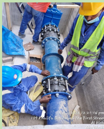
Chamber Fittings Assembly
