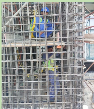
Inside Wall Steel Cage and Shutter preparation Work
