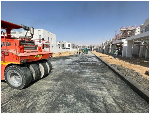
Road Base PTR Rolling and Compaction
