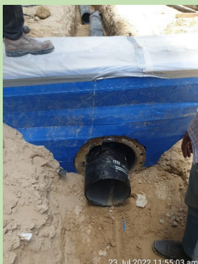
DI 300 Pipe passing through Sleeve
