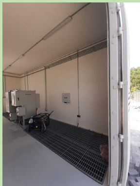
Floor Grating fixing
