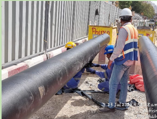
DI pipe rapping work and sleeve installation
