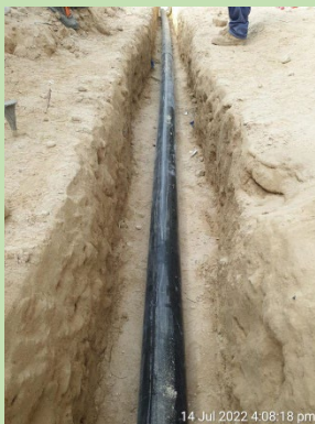
HDPE Pipe Laying in trench
