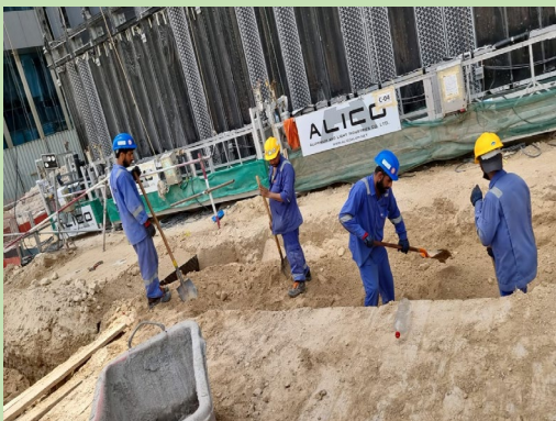
Trial Trench work to locate existing service
