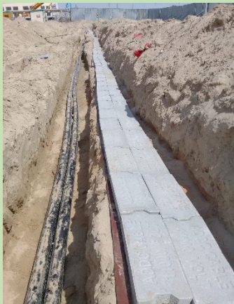
Electrical Protection Tiles and Cable Dressing with Warning Tape
