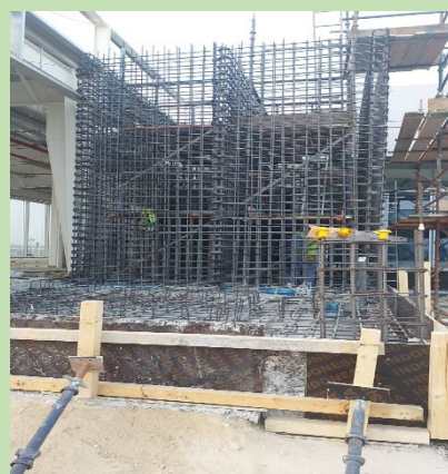
Raft Foundation, Steel Cage for wall
